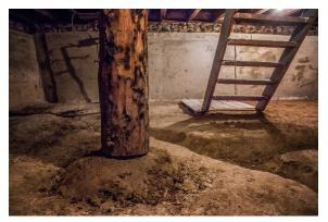
The basement was cut out of the ground and one large tree was cut down and used to support the center of the main floor. The house rested on a total of four such posts, with this main one resting on a partially buried bolder in the dirt floor. The chimney ran the entire height of the house, from the basement to the second floor.
